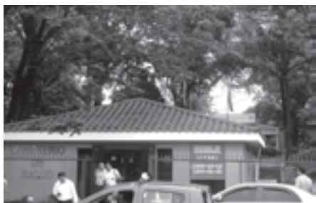
Entrance lodge to the ministry of health in Nicaragua
